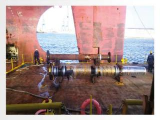
In parallel with the stern tube jobs the new shaft was received from the makers, then the propeller and the shaft were transferred to a pier where two cranes were hired.
