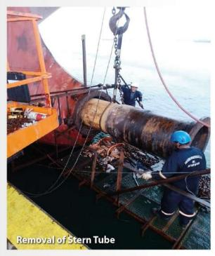
Talleres fabricated a structure to pull the forward end of the tail shaft with 2 jacks of 500 tons but is was not possible to remove the shaft, we concluded that the forward end of the tail shaft was seized to the stern tube so we decided to cut the forward end of the shaft with the flange to take the complete stern tube with the forward end of the damage tail shaft pulled aft through the stern casting.
