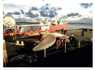
Finally, we installed the propeller, and the hydraulic nut performed the propeller push-up adjustment. The vessel was moved back to the anchorage to installation of the rope guard and the nut cap on the propeller and the inside continued the installation of the connecting bolts between the main engine flywheel, intermediate shaft, and propulsion shaft. We Installed all the hardware that was removed in the engine room to gain workspace.
