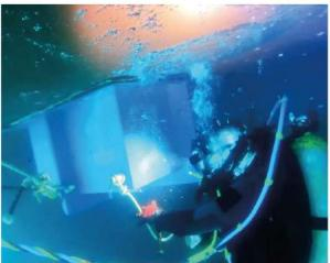
Many vessels face this issue due to the high sulfur content on the scrubber wash water, which is used to clean the fuel emissions to comply with International Maritime Organization (IMO) 2020 sulfur oxide emissions. Acidic water can create corrosion which results in a leak in the pipe, like in this case.
