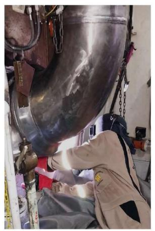
After the paint curina time class-approved welding was completed, divers proceeded to remove the cofferdam. Finally, the system was started, and the crew inspected that no leak was present. repairs were executed as class per requirements. Please call us 24/7 for any of your complex and challenging needs.
