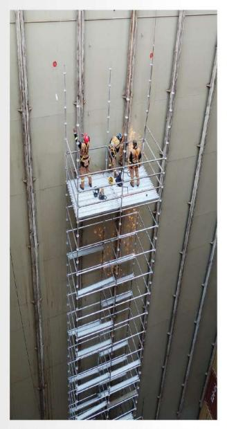
Tubular scaffolding is installed when you have a solid and secure platform which you can build upon to reach heights, plus job is accompanied by good weather (no rolling of the vessel).
