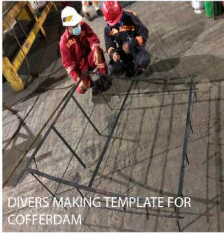
FABRICATION OF CUSTOM MADE COFFERDAM
