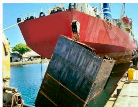
Full box cofferdam for rudder
